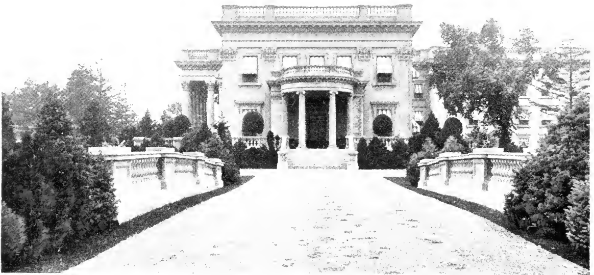
An elaborate conventional approach to the side entrance of a private residence. The stone bridge crosses a ravine.
